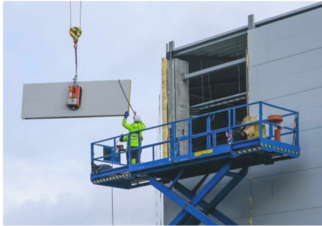
Figure 14. Prefabrication streamlines installation. Photograph courtesy of Zigmunds Dizgalvis.
