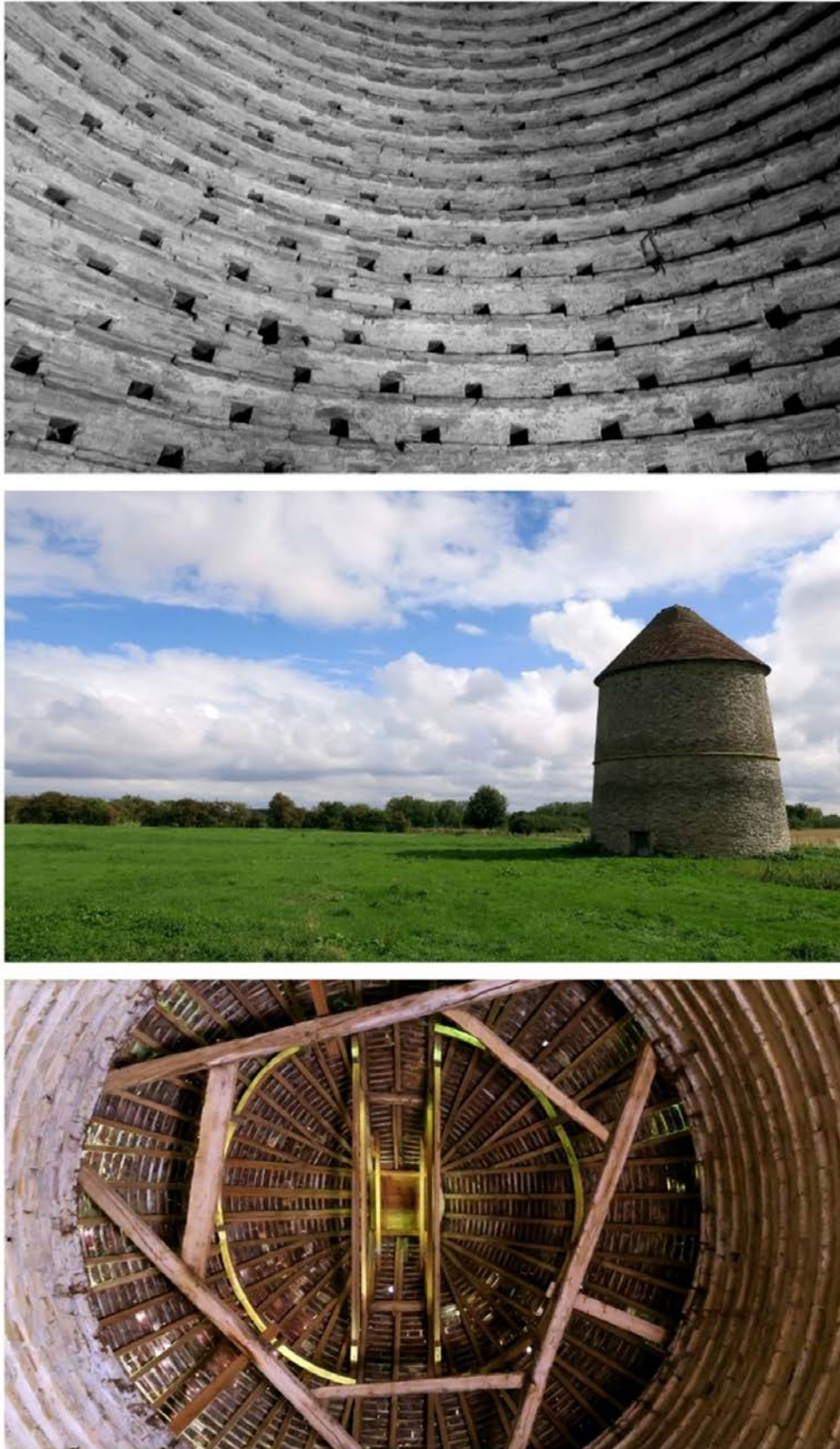
Figure 6. Sibthorpe Dovecote in Newark, Nottinghamshire (Cansu Curgen).
