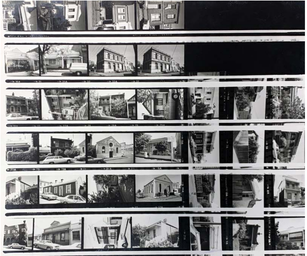
Figure 8. South Fitzroy conservation study: negatives, Jacobs Lewis Vines Architects, Dr M.B. Lewis, Fitzroy Urban Planning Office, 1979. Fitzroy Library, Local History Collection, LHREF BOX 10/ LH29/58.
